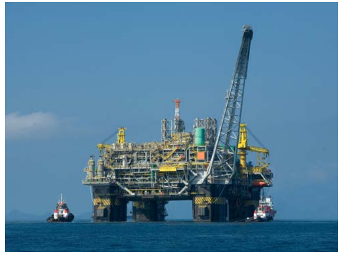
Currently used in off-shore platforms
